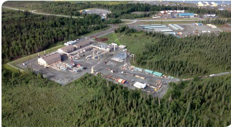
Cook Inlet Natural Gas Storage Project; Kenai, Alaska; in service since April 2012
